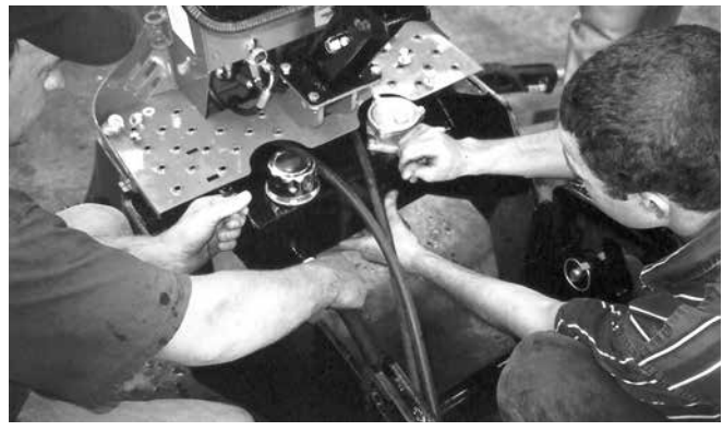
Fig. 5—Installing Reservoir in Backhoe Frame
